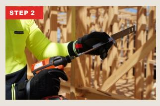
With the guide held in your hand place the screw in the nominated section with thumb located on the threaded part of the screw in a pistol grip hold.
