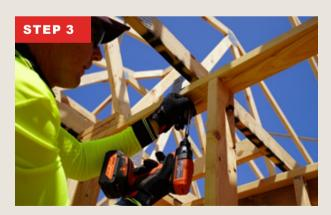
Then locate the truss as shown on the guide and proceed with installation.
