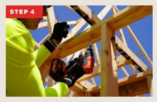
Remove the guide and continue to drive screw in one seamless movement, connection is complete when socket meets the top plate.
