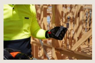
Use the supplied screw guide, so the screw is positioned in the correct location.
